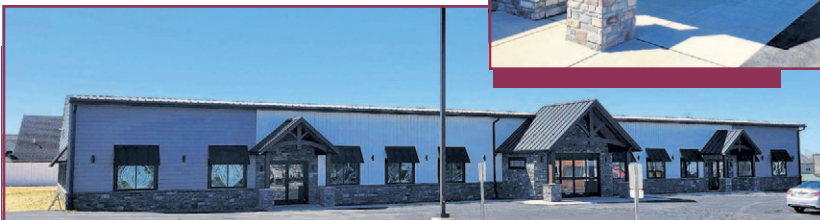
Commercial Building Remodel - (After)
