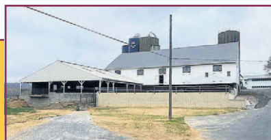
NRCS project in Penryn, PA (After)
