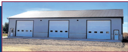
Ag Building 60' x 100' Equipment Storage
