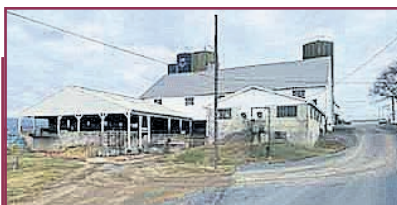
NRCS project in Penryn, PA (Before)
